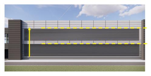
Parts of the façade where the escape stairs are located step out and are horizontally fixed, composite flat metal panels with mineral wool core, powder coated to a dark grey colour to help break up the massing of the building. The parts of the façade where the stair core pushes out also range in colour, getting lighter towards the external plant yard.
