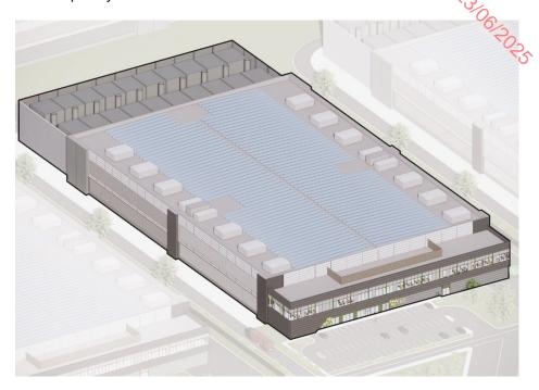
The external dimensions are approximately (including the external plant yard and to the widest point of the data hall facade) 184m x 91m. The façade along the data hall steps out, with changes in the colour of materials as well to help break up the massing.
